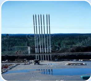
Thermosyphon Foundations for Buildings in Permafrost Regions
